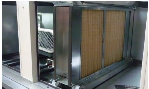
The Trane Air Cleaning System installed in an AHU.
