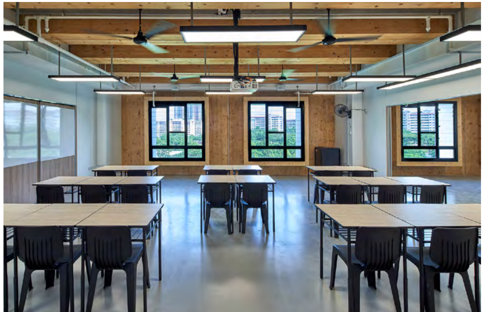
Using Mass Engineered Timber improved buildability and contributes to environmental sustainability. The use of wood for the interiors rekindles a connection with nature.
